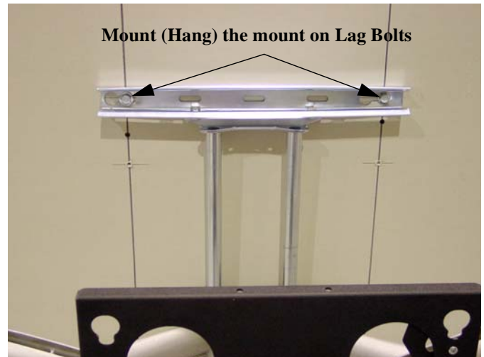
Figure 2. Mount mount on Lag Bolts
